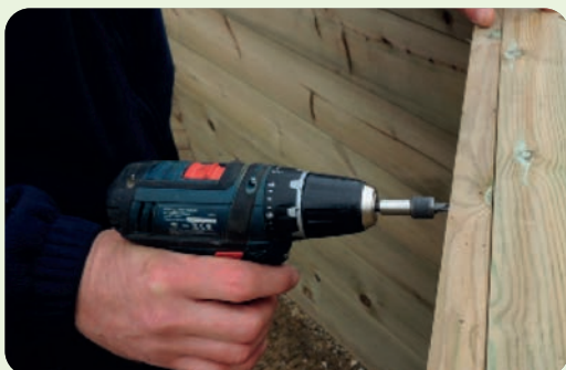
Fitting the Shelving Support
